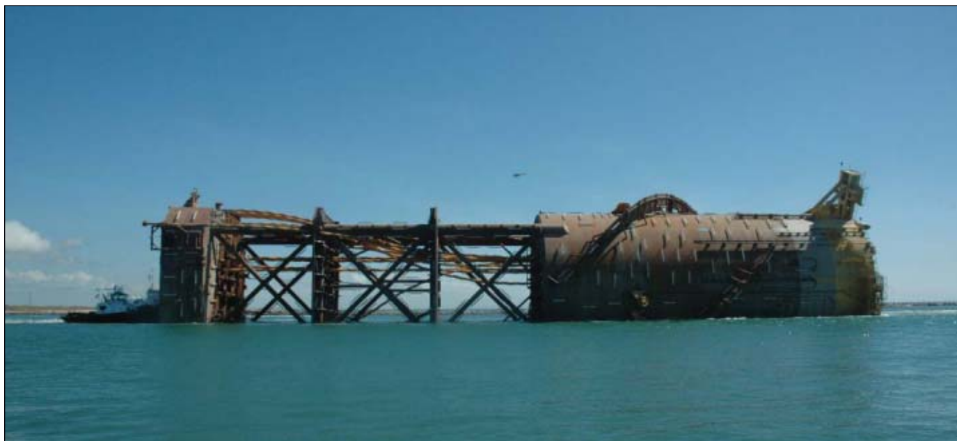
The Perdido spar drew about 42-ft draft as it sailed through the Aransas Pass jetties (Fig. 4; photo by Nina M. Rach).
