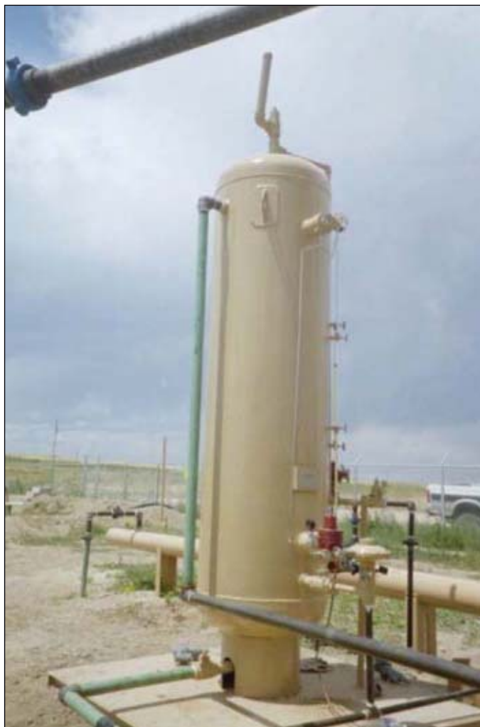
Field tests of this 36-in. diameter, 8-ft high surge bottle determined maximum oil production that the vessel could handle during a production cycle (Fig. 2).
