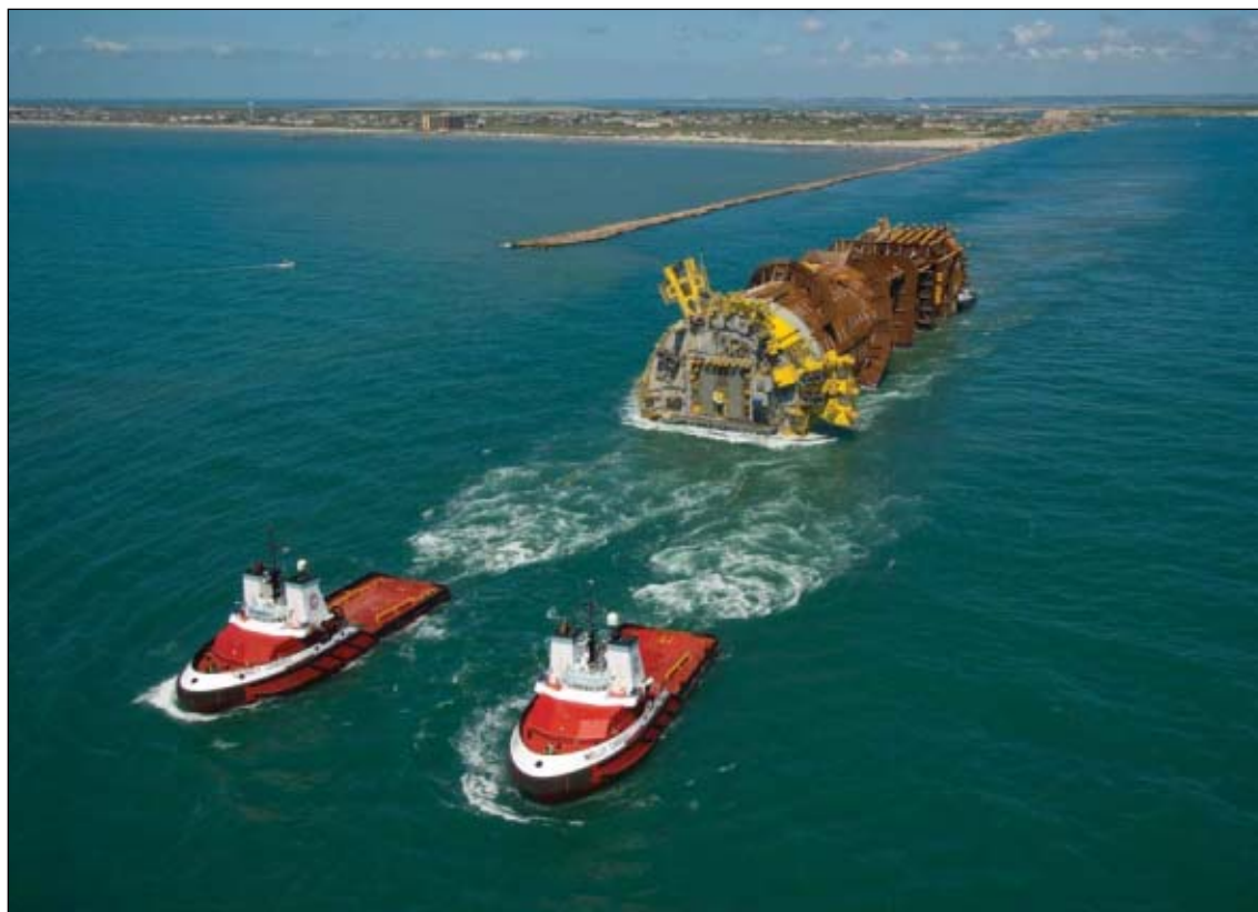
Otto Candies tugs pull the Perdido truss spar through the Aransas Pass jetties on Aug. 8, 2008, en route to Alaminos Canyon Block 857 (Fig. 1; photo from Shell).
