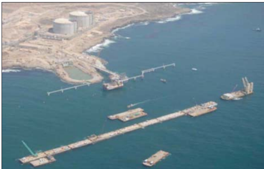
Onshore LNG import terminals might require a breakwater such as used by Semptra at its Costa Azul terminal in Baja California, Mexico. The absence of a breakwater could lead to manifold motions extending beyond the working range of the arms unloading the ship (Fig. 2).
