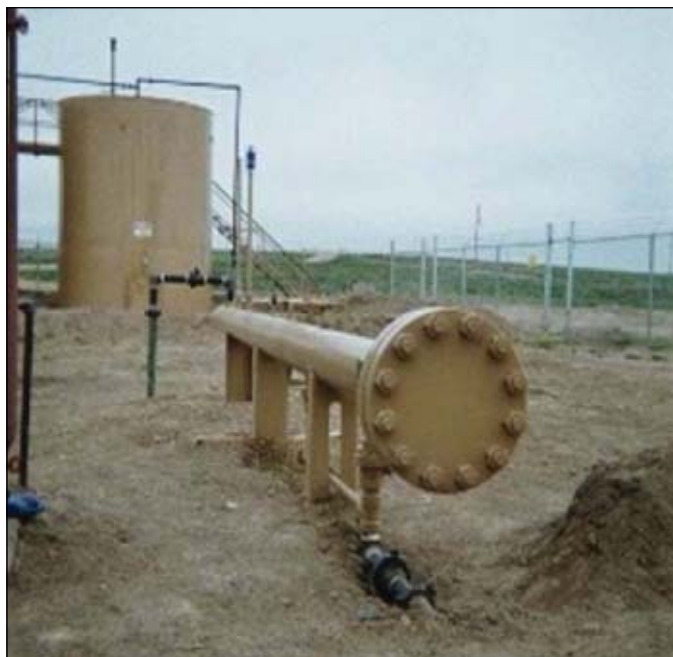
Personnel will test this prototype slug catcher when oil production peak rates at the site decrease to about 1 bbl/cycle (Fig. 4).
