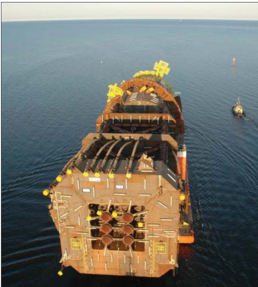
The Perdido spar sails from Finland in May 2008 in a dry lift aboard Dockwise Shipping BV's Mighty Servant I . The tops of the six risers will attach to the bottom of the spar's soft tank, shown above (Fig. 3; photo from Shell).
